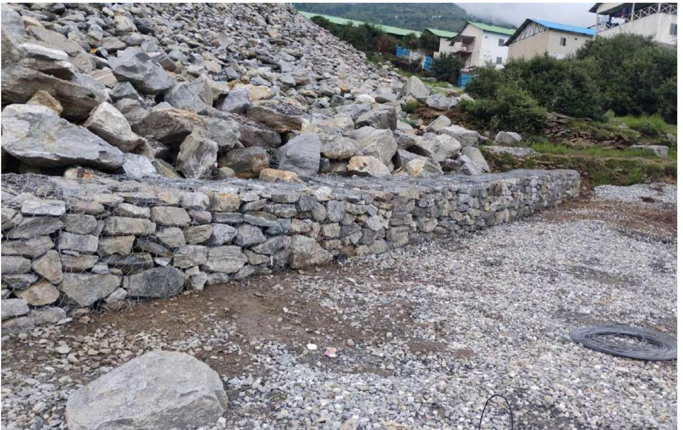
**Photographs Showing Toe Protection work for stacked muck near Joshana Village
