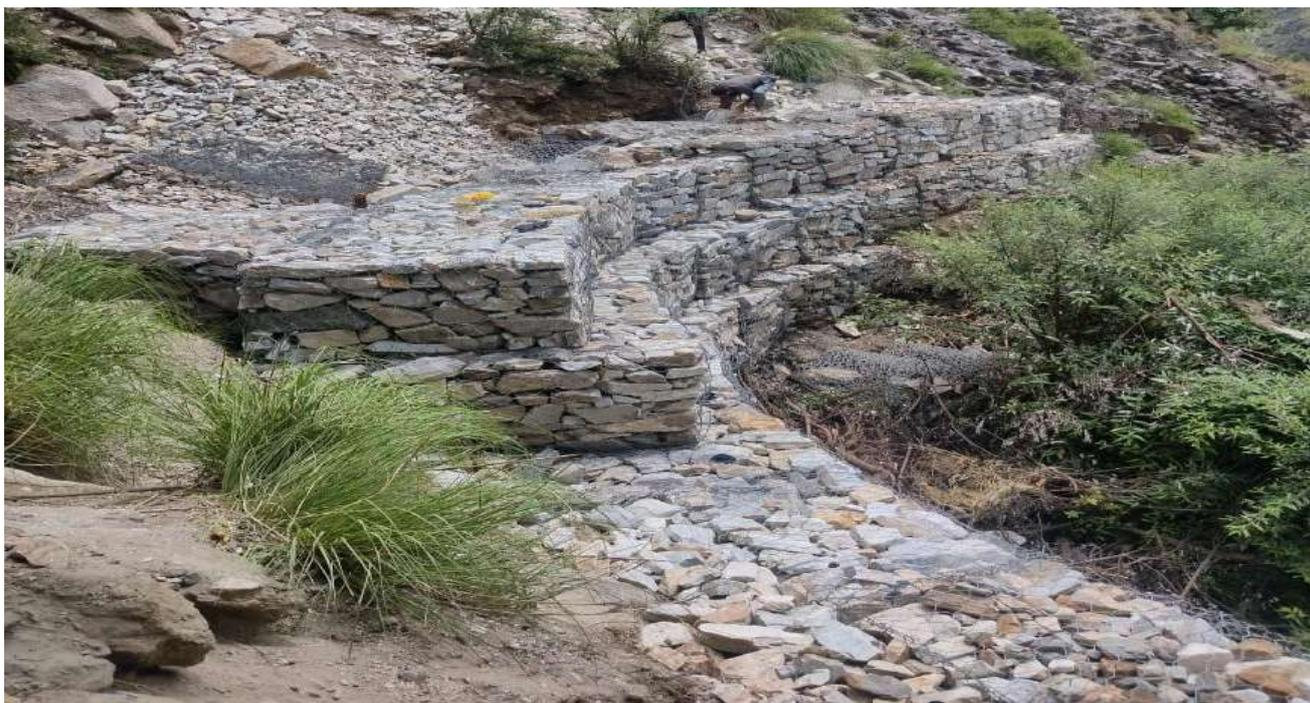
**Photographs Showing Toe Protection work for stacked muck near Hasti.**
