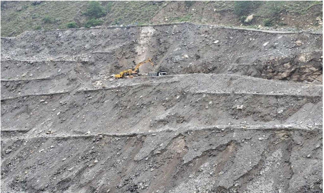
**Photographs Showing Removal of Muck from Zone-1 (Right Bank Downstream)**
